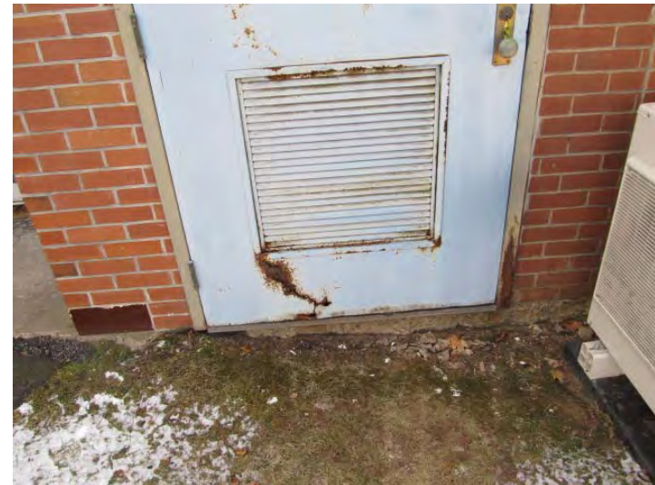
Rust-damaged service door at community building mechanical room
