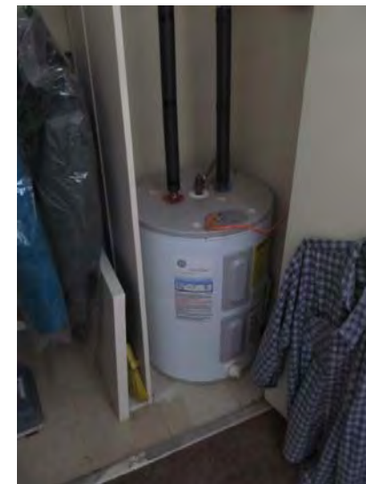
Each unit has an electric, storage-type, domestic hot water tank
