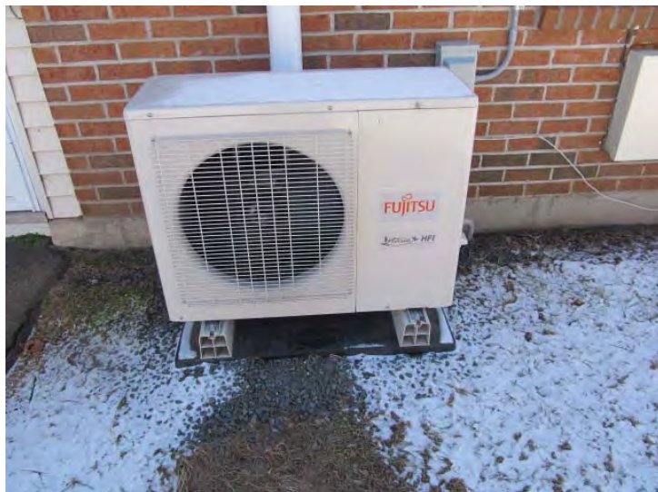
Typical exterior condenser for heat pumps that were recently installed in all units
