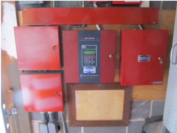
Fully addressable fire alarm control panel has been updated in recent years
