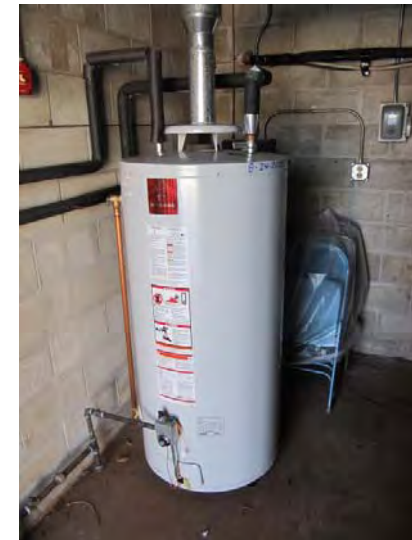
Natural gas-fired domestic hot water tank for community building
