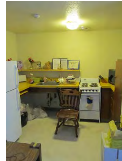
Handicap accessible unit kitchens include knee clearance space under the countertop
