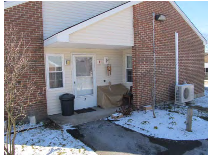
Brick veneer, vinyl siding, windows, and doors all in good overall condition
